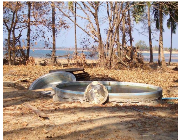
Damage to the Naucrates turtle project tanks after the tsunami. Photo by Emma Dilkes
